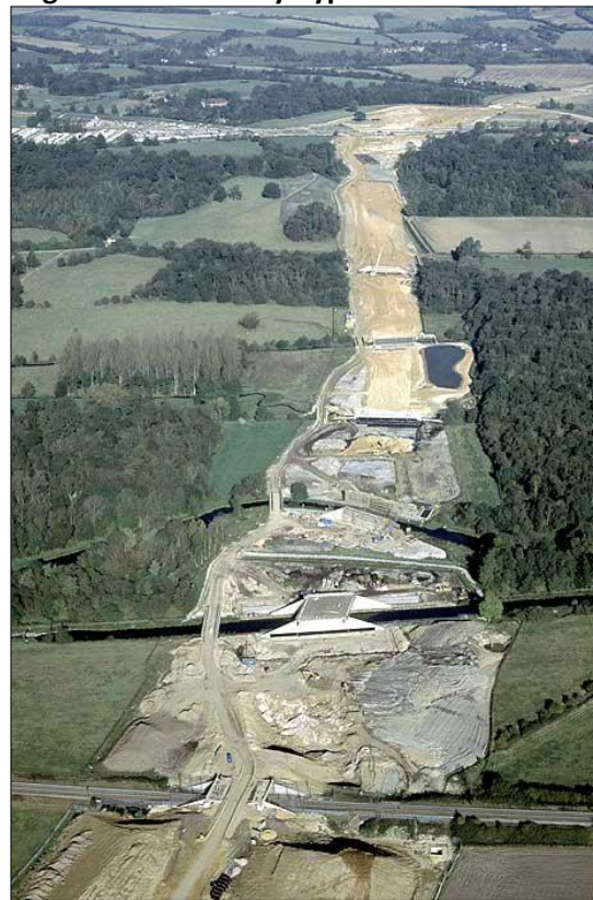
Figure 1.2: Newbury Bypass construction
