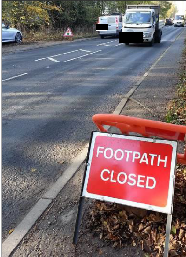
Figure 10.4: Heavy traffic and inadequate provision for cyclists and pedestrians on the former A120
