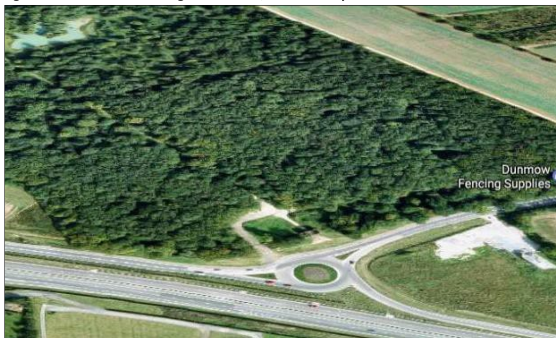
Figure 10.5: Aerial view of High Wood SSSI, where cut by A120
